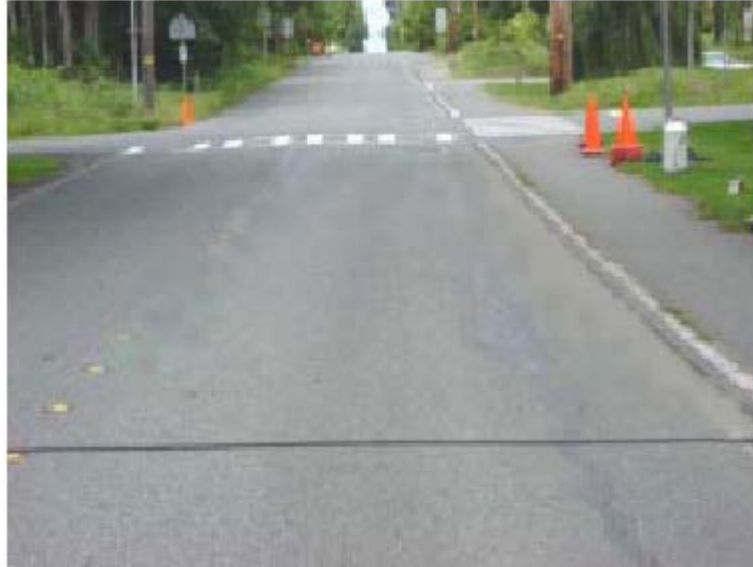
Before instalation in Edmonds, WA (U.S.A.)
